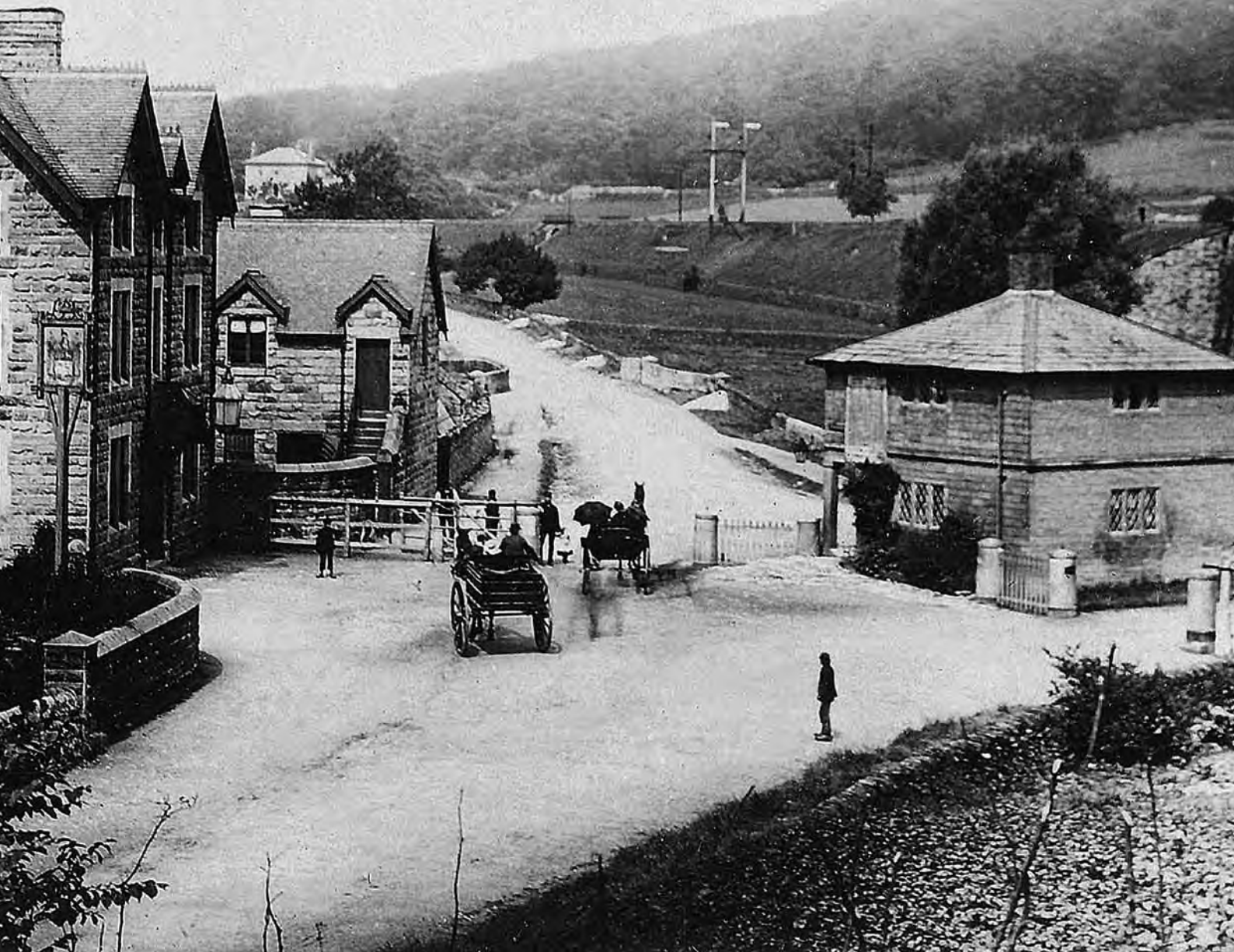
Toll house and gate at Ambergate, c.1880
