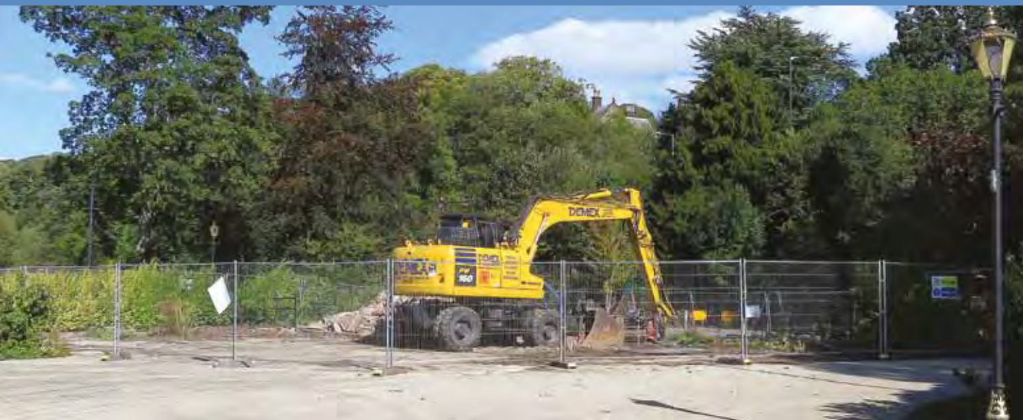
Demolition of the old tearooms, Belper River Gardens
