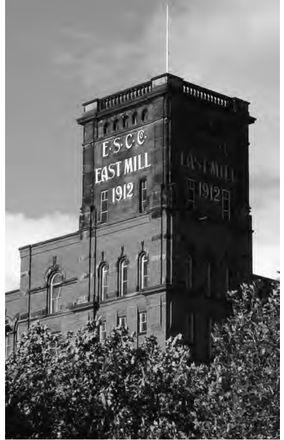
Belper's East Mill water tower
