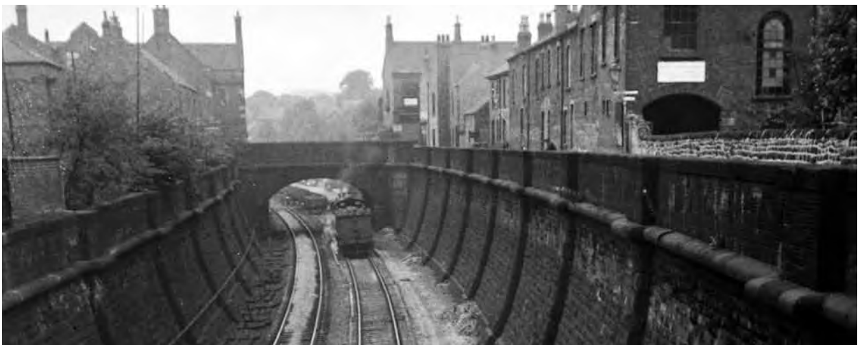
Belper railway cutting, 1947
