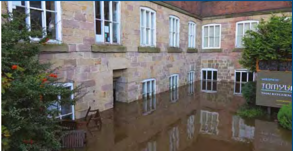
Flooding at the Belper Mill Complex, 2019
